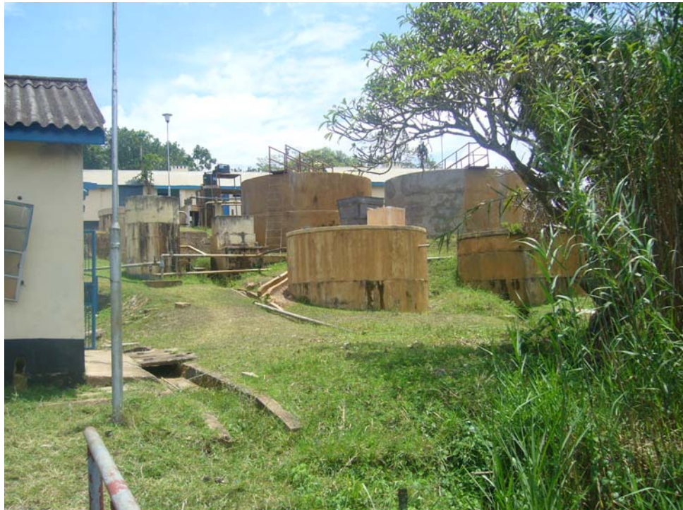
Fig. 3 – Bondo Water Supply intake and treatment works at Yala River
