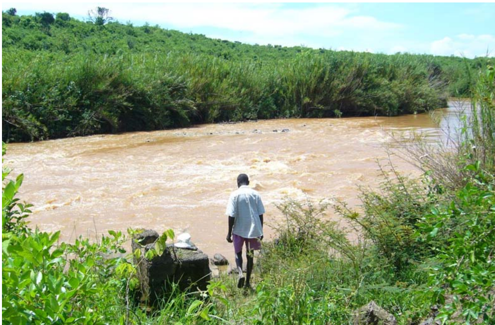
North Sakwa – what is left of the intake structure
