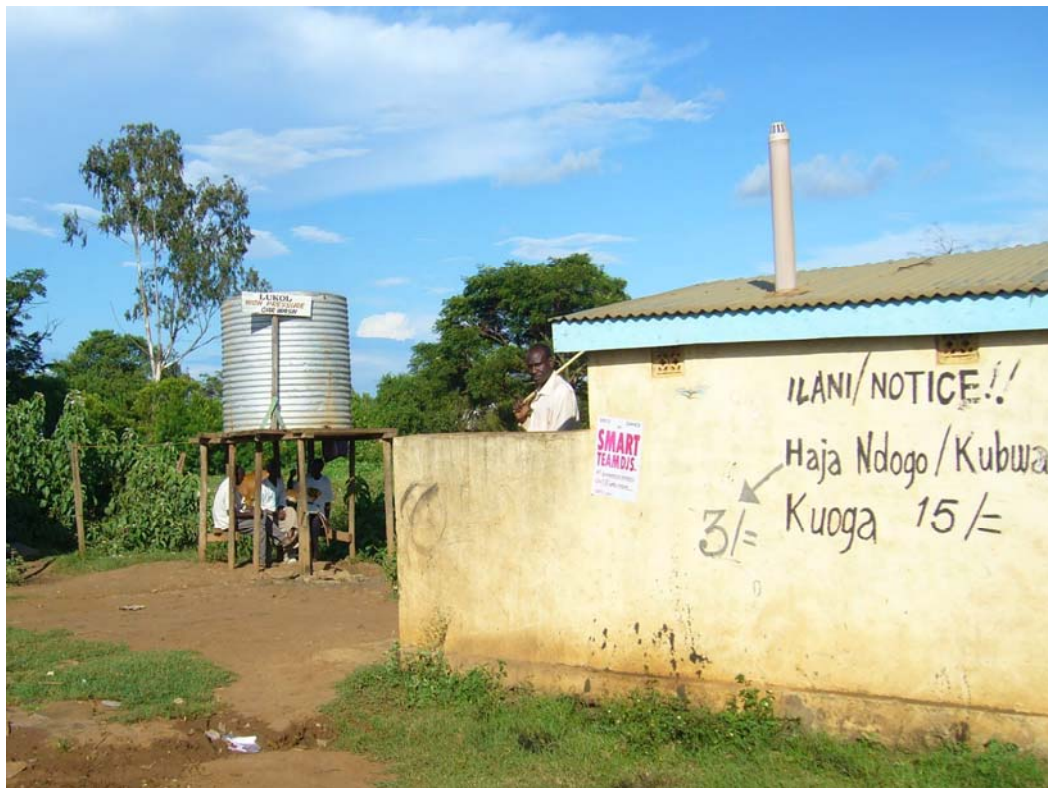
Public stand pipe, car wash (high pressure!) and public toilet at bus station
