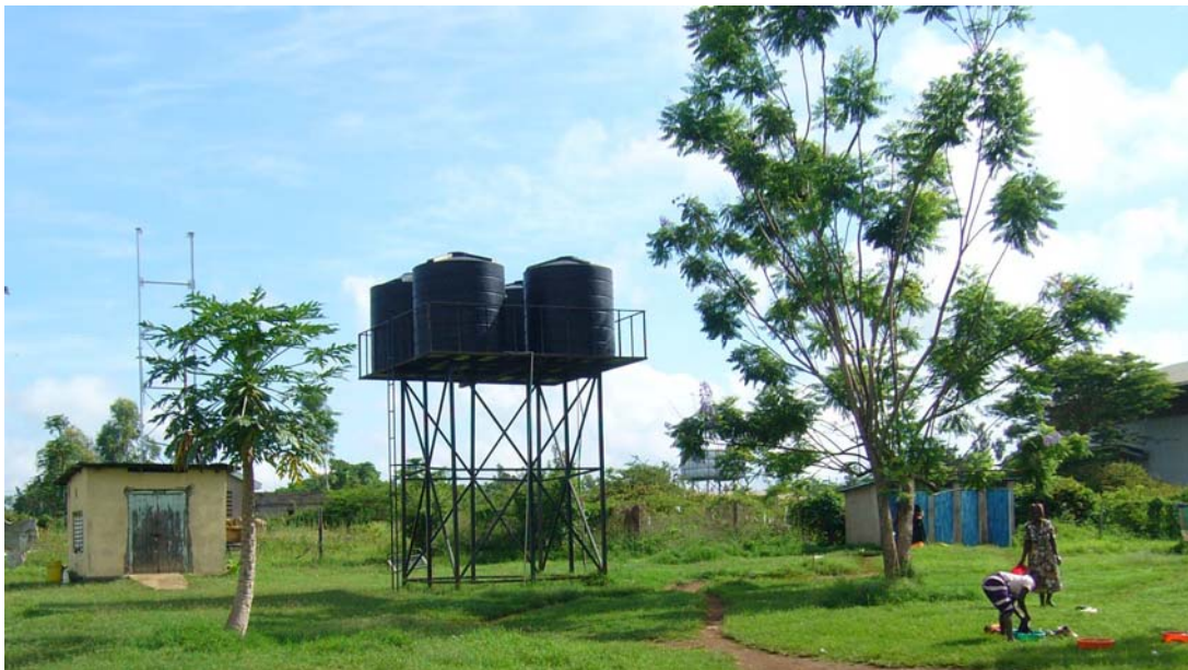
Water storage at Bondo District Hospital; pit latrines in right-hand corner.
