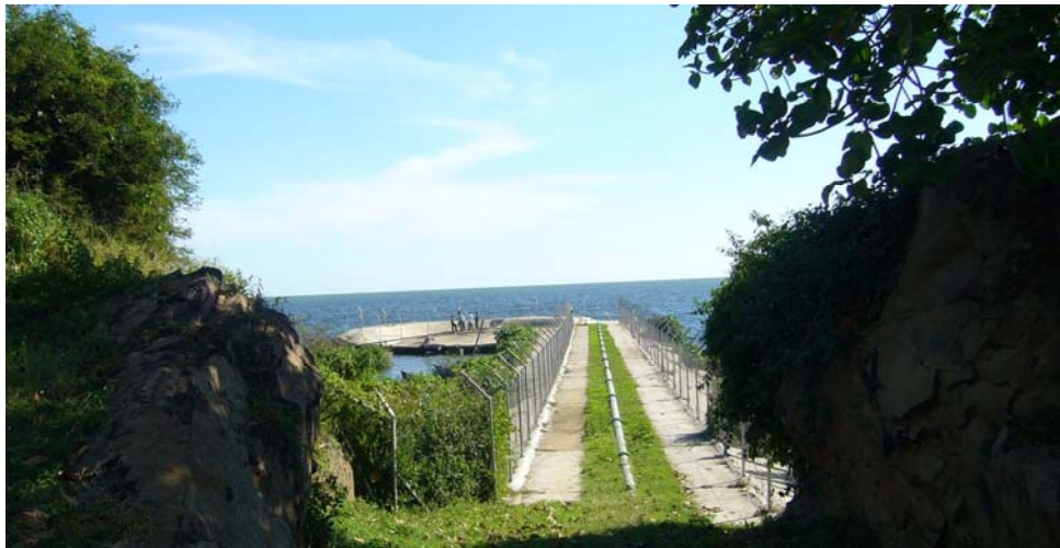
Intake structure for South Sakwa w/s
